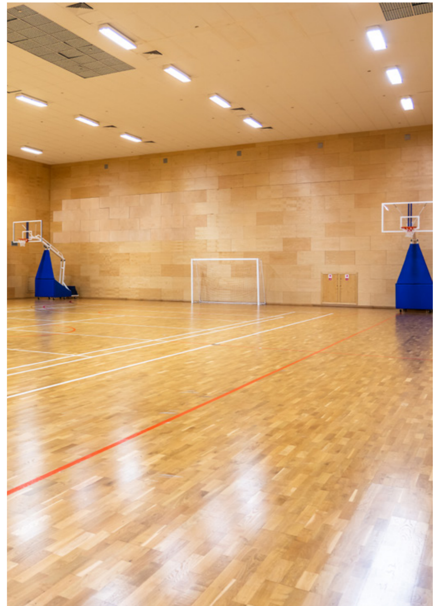
Application of Arena LED.
